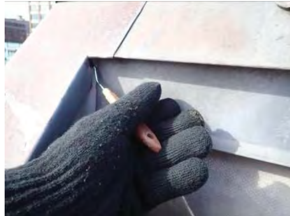
Photo No. 13 - Photo depicts a tactile probe inserted into an opening at the sheet metal eave edge flashing-to-membrane-lined gutter intersection. This condition was observed in the majority of the areas accessed and appears to be a typical condition – all of which are in need of backer rod and sealant and properly formed, fit, and secured sheet metal corner closures.
