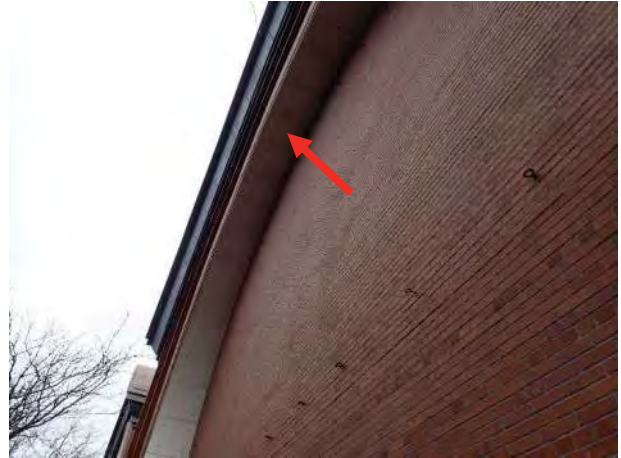
Photo No. 114 - Overview of aluminum cladding panels at small soffit area at repeating arched bay at the West Elevation.
