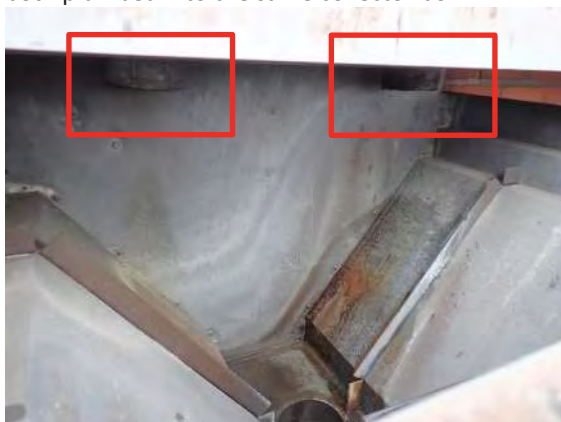
Photo No. 42 - View of the primary drain and the secondary overflow drain both plumbed into the same collector box.
