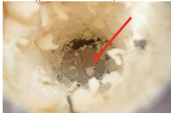
Photo No. 27 - Depicts existing concrete roof deck observed at test opening. No vapor retarder was observed at the area of the test opening. The black material, located just above the red arrow down in the test opening, is the bottom-side recycled-cardboard facer of the single-layer of rigid-roof insulation.
