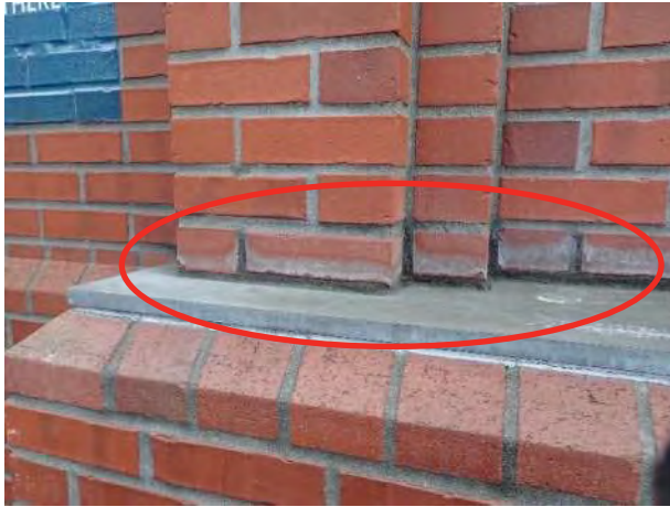
Photo No. 52 - View of moisture-migration related staining at archway base locations at the West Elevation of the Museum above the steel base plates that do not have proper slope to drain.
