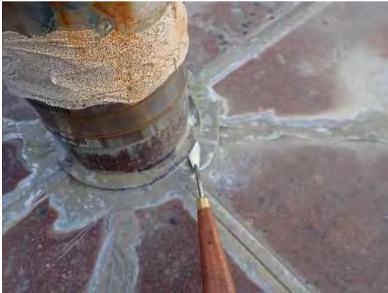
Photo No. 6 - Depicts broken solder joints at the sheet metal flashing around a fall protection anchor at the apex of the steep-slope roof area, which needs to be repaired and flashed over.
