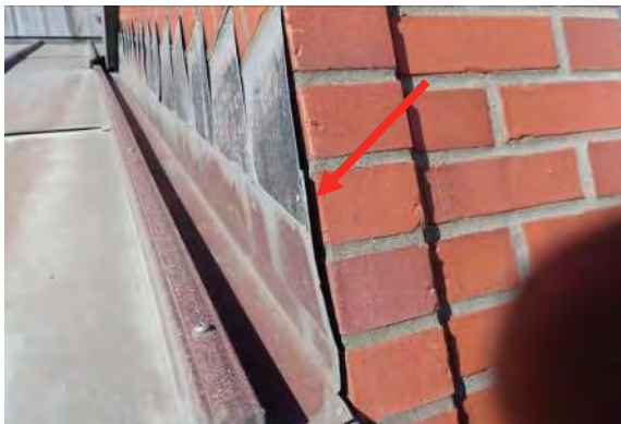
Photo No. 22 - Photo depicts weather-exposed opening between the sheet metal roof-to-rising wall flashing that extends up onto the brick veneer at the South Elevation of the Anthem Café Dormer. Incompletely terminated and unclosed sheet metal components, and the lack of a diverter flashing leaves this area vulnerable to wind-driven rain, and snow- and ice-melt moisture intrusion.
