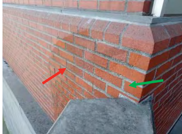
Photo No. 90 - Depicts the limited surface moisture testing at the North Elevation that revealed localized deficiencies in the clear siloxane-based water repellent, indicating that portions of the water-repellant have reached the end of their useful service life, and are allowing moisture to penetrate into the surface of masonry components. 'Dry' appearing areas of coating at green arrow are more in-tact than the 'wet' appearing area at the red arrow.
