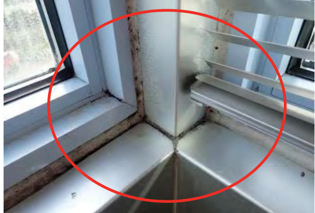
Photo No. 100 - View of black and dark-colored fungal growth (e.g., mold) stained silicone sealant joints at the interior, as well as water droplets on the aluminum frame due to condensation forming on aluminum frame.
