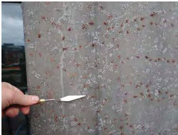
Photo No. 85 - View of biological growth and staining observed on the exposed concrete walls at the East Elevation likely from crawling vines on that side of the Building.
