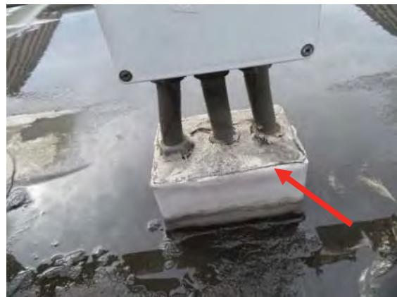
Photo No. 31 - The pourable sealant installed as the electrical-conduit penetrations' "flashings" was observed to be aged, failing, and in numerous areas cracking and shrinking away from the perimeter of the pitch-pan, leaving the area vulnerable to moisture intrusion.
