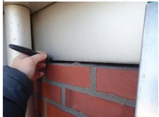
Photo No. 70 - View of the errantly left gap at the top of the brick veneer wall, at the East Elevation of the Anthem Café, which has been susceptible to water migration. This open joint should receive a backer rod and sealant joint to close this vulnerable location.
