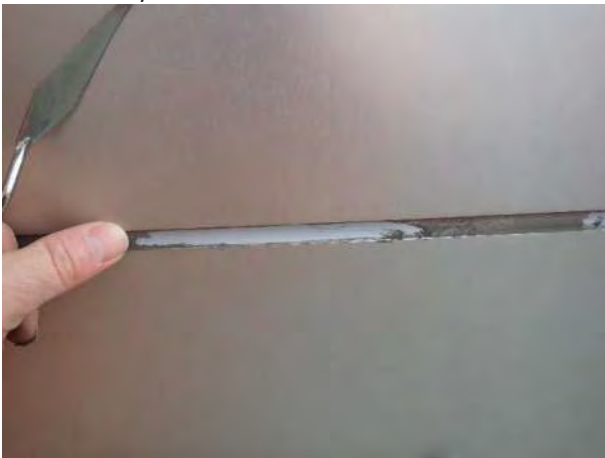
Photo No. 115 - View of typical silicone sealant joint at aluminum panel butt joint intersections. The majority of the sealant is in relatively good condition and functioning as intended.
