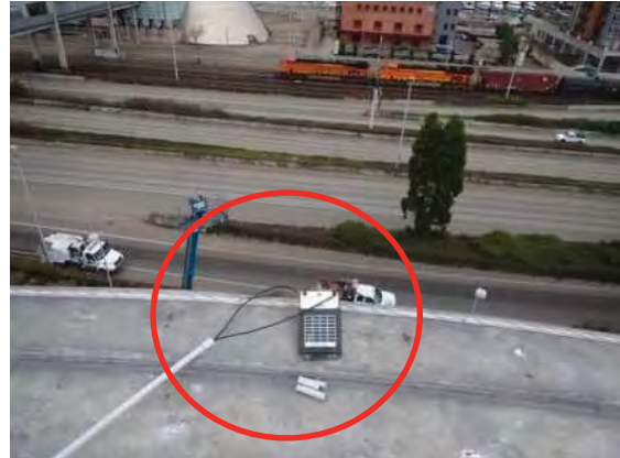
Photo No. 11 - Photo depicts loose electrical equipment and components at the apex of the steep-slope barrel roof area on the east side of the building. The bird deterrent system should be repaired, secured, or removed soon.
