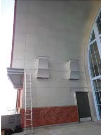
Photo No. 113 - Overview of aluminum cladding panels which are mechanically attached and comprise the exposed soffit areas of the archways, both large and small. This photo depicts large soffit area outside of Main Entry at the North Elevation.
