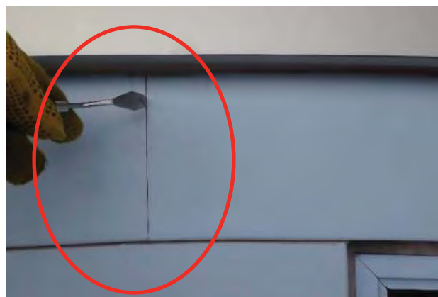
Photo No. 98 - View of open .125-inch thick aluminum panel joinery associated with storefront window systems observed at the West Elevation arched windows. Careful tactile probing suggested a backer plate is present, as detected behind the open joint.
