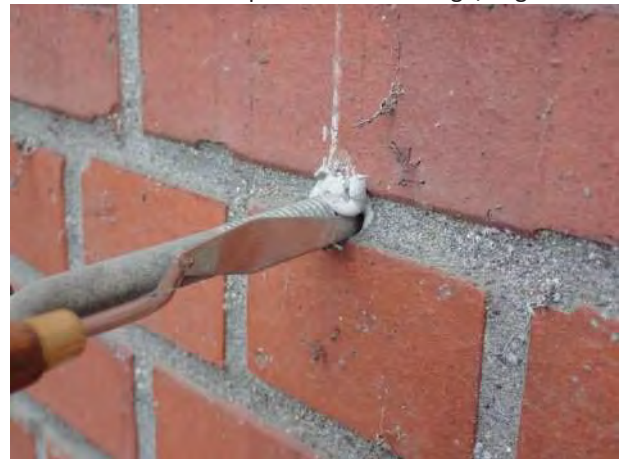
Photo No. 51 - Depicts epoxy set eye-bolt locations through the brick veneer that are not fully sealed and are open to leakage and water migration into wall.
