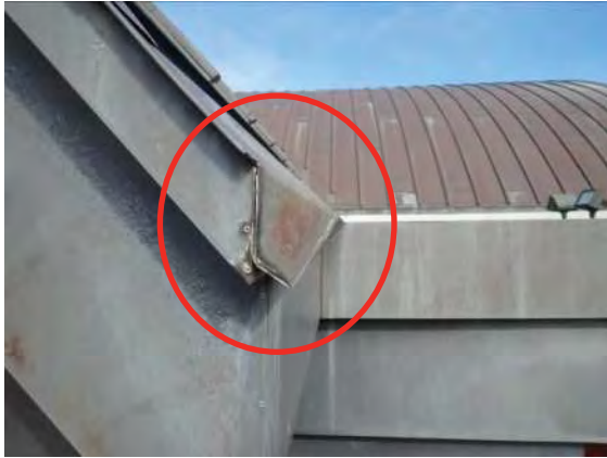
Photo No. 16 - Photo depicts aged and failed sealant joint at the roof's perimeter rake edge flashing-to-sheet metal gutter flashing intersection.
