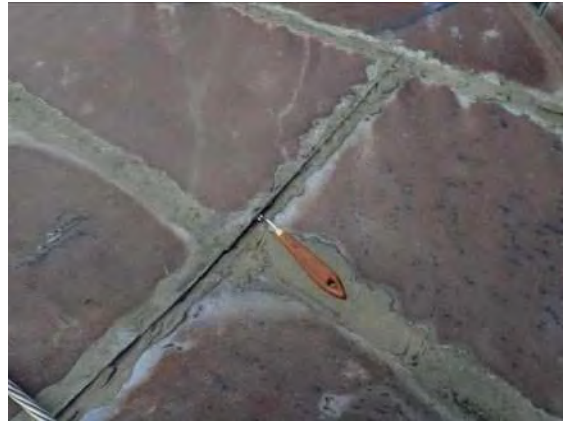
Photo No. 7 - Depicts probe inserted into a broken solder joint near the apex of the sheet metal roof area, this location was in a more heavily trafficked portion of the roof area and may have been caused by repeated roof maintenance traffic applying pressure to the solder joint, rather than stepping over and past the joint.
