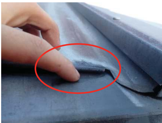
Photo No. 20 - Photo where staining and moisture was visible, apparently exuding out from between sheet metal components immediately down-slope of the problematic dormer-to-main field of roof intersection.
