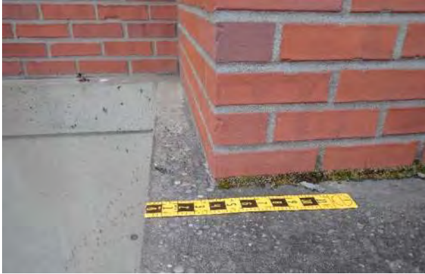
Photo No. 87 - View of skyward-facing concrete ledges that are susceptible to water pooling, the growth of moss, and other staining, as well as moisture migration, as evidenced by the degree of moss growth depicted in this photo.
