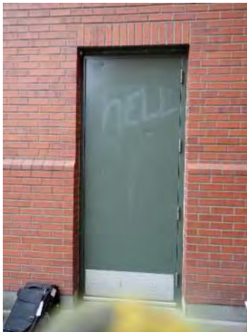
Photo No. 61 - View of typical Hollow Metal Door (HMD) and location of bedding-mortar joints at perimeters of door frame that are cracking due to differential movement.
