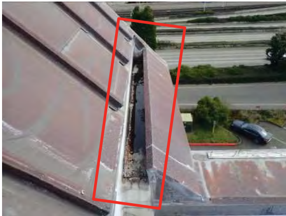
Photo No. 32 - Photo depicts water ponding within an exemplar membrane-lined built-in gutter adjacent a low-slope roof area. As the water level indicates, the gutter is improperly sloped -- sloping away from the draining end rather than towards the gutter exit.
