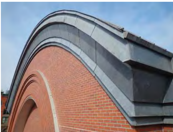
Photo No. 111 - Overview of sheet metal cornice at South Elevation. Although some staining was observed on the surface of the metal much of the staining appears to be related to roof-edge drainage issues.
