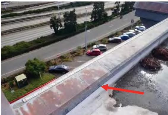
Photo No. 36 - Red arrow indicates the sheet metal, counterflashing which engages into the roof-side hem of the parapet’s sheet metal coping flashing. The hem was observed to be unevenly engaged at numerous locations, and in some cases had been attempted to be secured with rivets.
