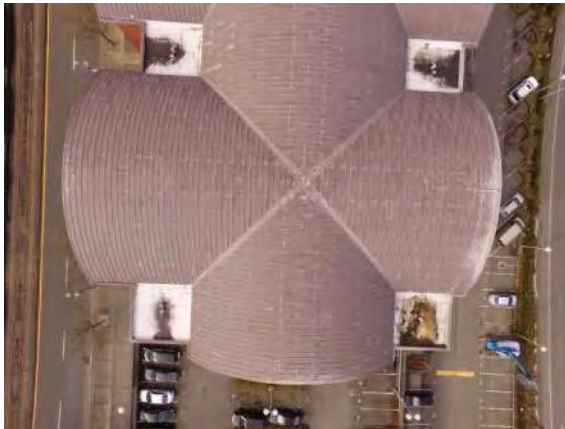
Photo No. 38 - Drone overview of the South Portion of the Museum's Main Roof illustrates extensive areas of ponding and staining observed on the low-slope roof areas, partly due to clogging of the roof-side drain strainers.
