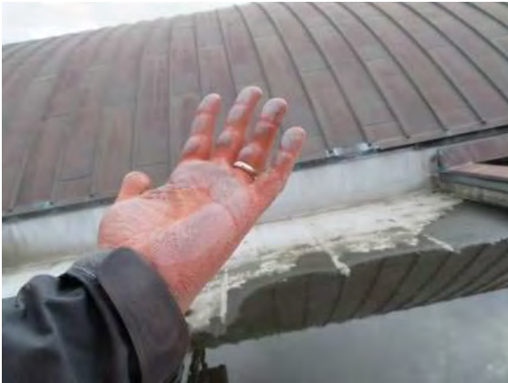
Photo No. 28 - Chalky residue visible on BET&R's Survey Technician's hand after light hand pressure was placed on the existing Hypalon roof membrane. In general, the oxidized chalky surface indicates that the primary top surface of the roof membrane is aged and weathered.
