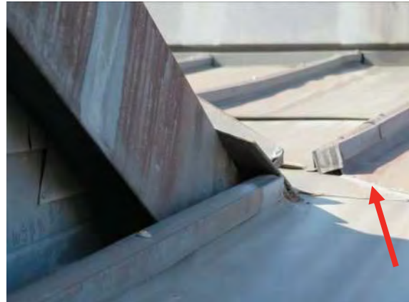
Photo No. 19 - Depicts close view from a different angle of the sheet metal apex flashing-to-main roof area transition. Water was observed behind and beneath the sheet metal roofing and flashing downslope of this location, indicating that this vulnerable intersection is allowing moisture into the roof system.
