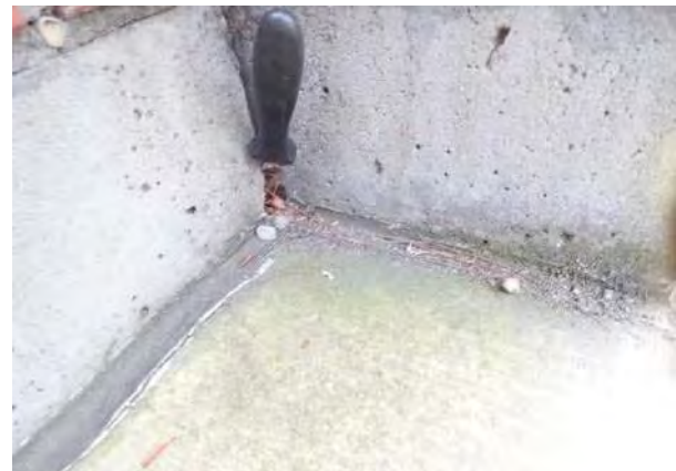
Photo No. 120 - View of flat probe inserted in to the failed and open inside corner of a different sealant joint at the expansion joint.
