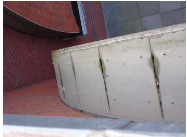
Photo No. 84 - Another view of decorative aluminum panels at large archway tops, as observed along the two arches near the main entry at the North Elevation, and related moss growth and staining associated with the vulnerable gaps between the 0.50-inch thick aluminum decorative cladding panels, which essentially are serving as roofing and cladding over the arched masonry.
