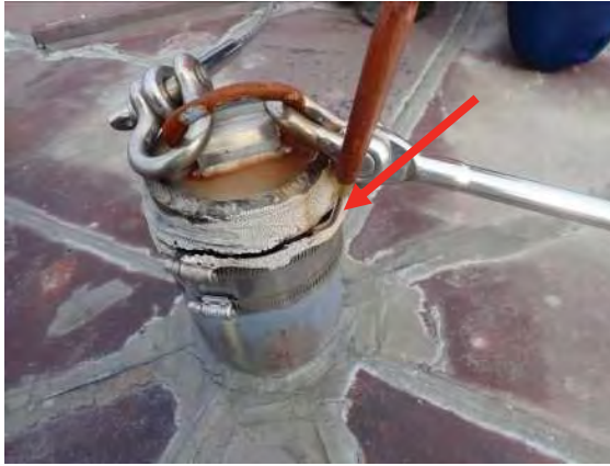
Photo No. 8 - Depicts a round-nosed probe inserted into a cracked and failed sealant joint at the fall protection anchor at the south end of the steep-slope roof area.
