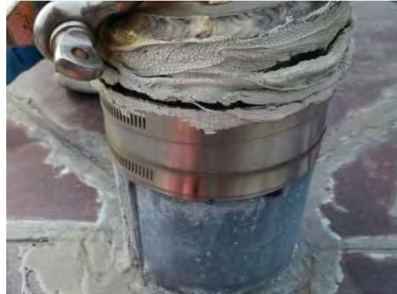
Photo No. 9 - Depicts weathered, degraded, crazed and cracked sealant joint at a fall protection anchor on the steep-slope roof area.
