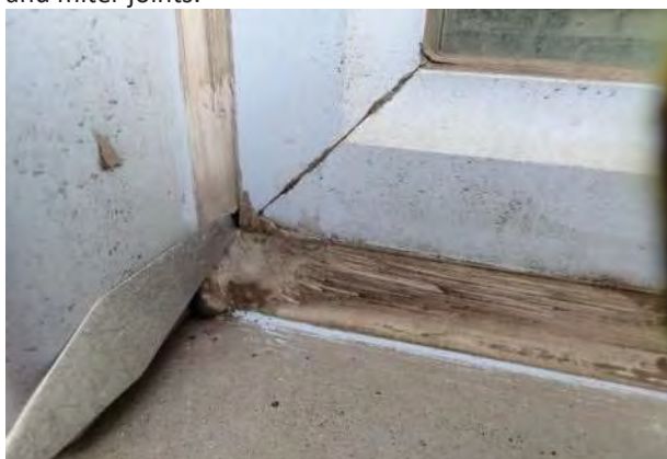
Photo No. 97 - View of small sealant failure at jamb-to-sill intersection. Although minor locations of failed sealant were observed, the majority of the sealant appears to be in serviceable conditions.
