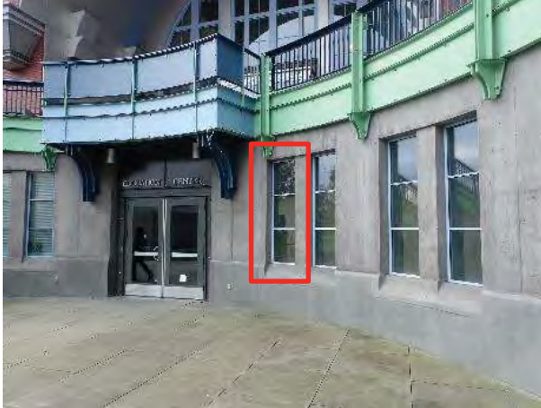
Photo No. 105 - Overview depicts area where typical extruded-aluminum framed, double-glazed window unit is set in cast-in-place concrete opening. The superimposed red box depicts the specific window unit that was tested. Sealant joints generally appeared satisfactorily -bonded and did not exhibit adhesive nor cohesive failure, surface chalking, crazing, or other visible signs of degradation. This window unit did not allow any water to the interior of the building during the test, and was determined to 'pass the controlled-spray diagnostic water test.'
