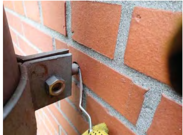
Photo No. 49 - View of typical bracket sleeve connection for downspouts through the brick veneer that is unsealed and open to water leakage/migration.
