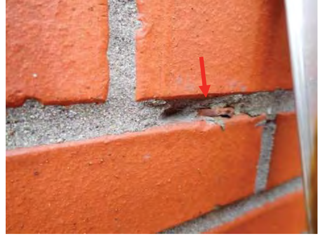
Photo No. 66 - View of scaffolding tie-back embedded in mortar joint and causing isolated spalling as it corrodes.
