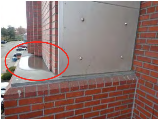
Photo No. 54 - View of negative shelf slope and resultant pooling water discovered at steel plate archway bases contributing to the staining and moisture absorption issues at the brick masonry.
