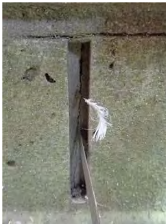
Photo No. 121 - View of flat probe inserted into the wider-than-hairline crack at the plinth control joint.
