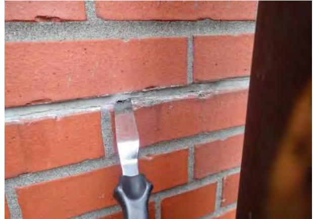
Photo No. 45 - View of flat probe inserted into an adhesively failed sealant joint at brick masonry veneer floor-line joint. This is a typical condition.
