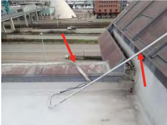
Photo No. 10 - Photo depicts displaced and progressively detaching electrified bird deterrent strips and loose and damaged plastic conduit at the steep-slope-to-low-slope transition at the northeast corner of the building. The bird deterrent system should be repaired, secured, or removed soon.
