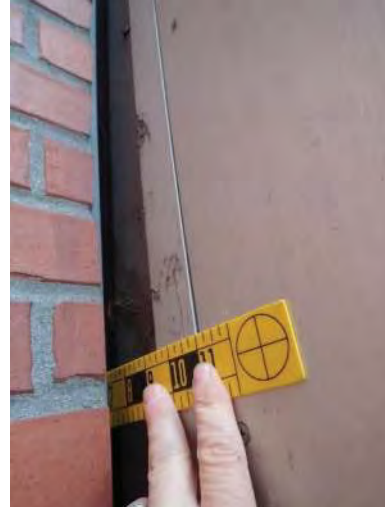
Photo No. 78 - Ruler inserted into void at brick veneer ledger angle to archway panel cladding at adjacent to the Main Entry Area, which is open to water leakage into the wall assembly, which may be causing hidden degradation and damage to underlying components.
