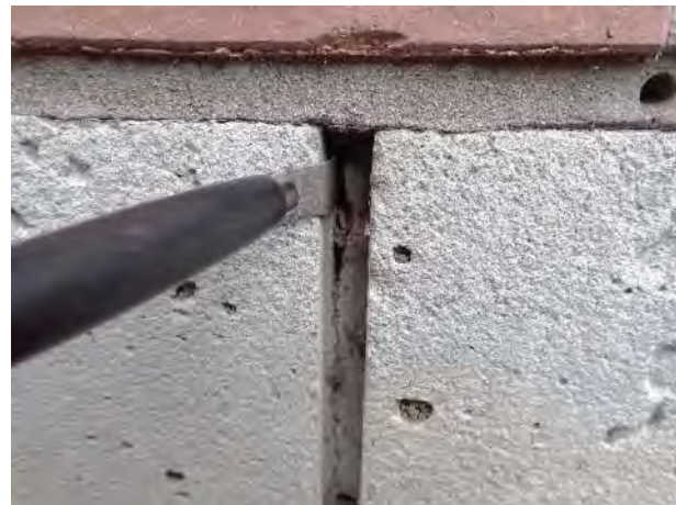
Photo No. 122 - Close-up view of cohesively failed and open control joint at precast concrete plinth.
