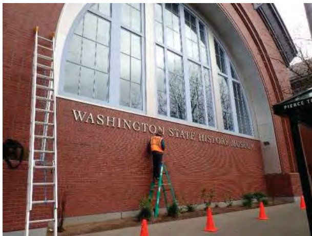
Photo No. 95 - Overview of large storefront type windows at the west elevation of the Museum. The window system observed at this location is dual pane window system set into extruded-aluminum frames surrounded by extruded aluminum trim, with silicone sealant joints at transitions and miter joints.
