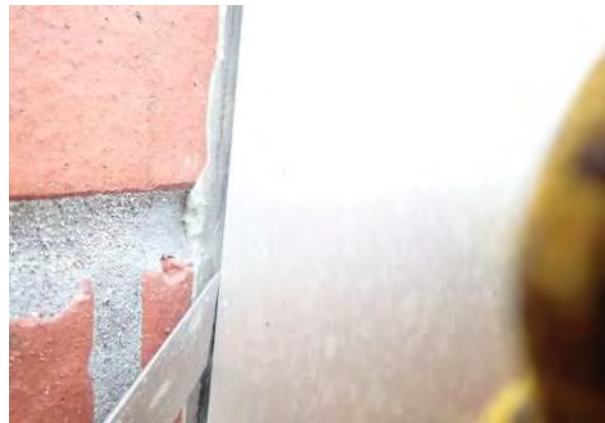
Photo No. 47 - Depicts weathered, aged, and failing sealant at the brick masonry veneer-to-decorative archway aluminum panel intersection. Of note, the Project Record Drawings do not show a sealant joint at this location. It is possible the sealant may have been installed during the brick masonry cleaning and sealing project of 2002.
