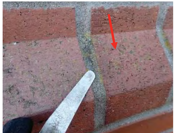
Photo No. 55 - View of yellowish-green colored moss or lichen growing on the chamfered, skyward-facing rowlock course, indicating that numerous mortar joints are showing signs of weathering, and getting a bit porous, and capable of holding a bit of moisture in their slightly eroded surface, which are beginning to support some organic growth.
