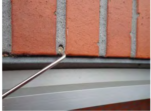
Photo No. 64 - Close-up of plugged weep tube discovered at a brick archway. In areas, the numerous clogged weep tubes may be adding to the moisture absorption and resultant staining observed at portions of the brick veneer cladding.
