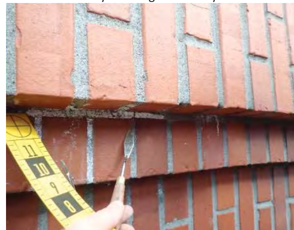
Photo No. 58 - Closer view of relatively heavy efflorescence deposits along the underside of archway brick detail.
