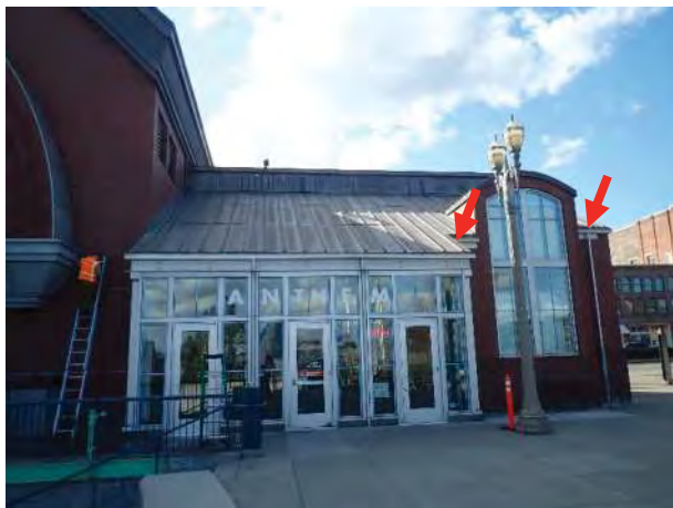
Photo No. 69 - Overview of East Elevation of Anthem Café and location of open brick veneer cladding transition at head of wall.
