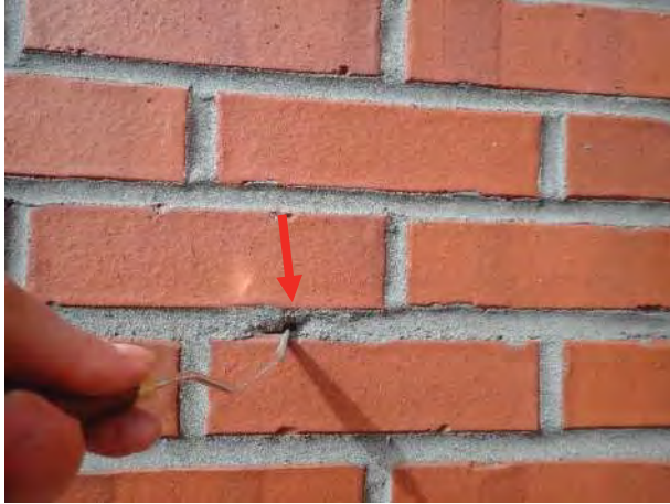
Photo No. 65 - View of scaffolding tie-back, carelessly left embedded in mortar joint, and causing mortar spalling as the steel corrodes.
