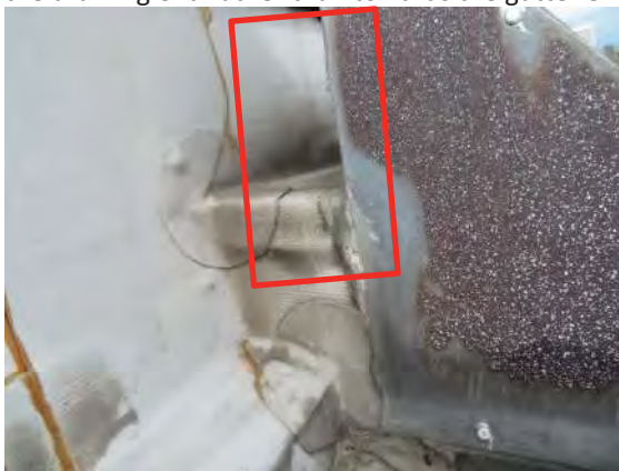
Photo No. 34 - Photo depicts area where either a sloped “kick in” flashing should be installed, or better yet a re-sloping of the gutter trough during the upcoming reroofing so as to direct water away from the vulnerable parapet-to-gutter termination intersection.
