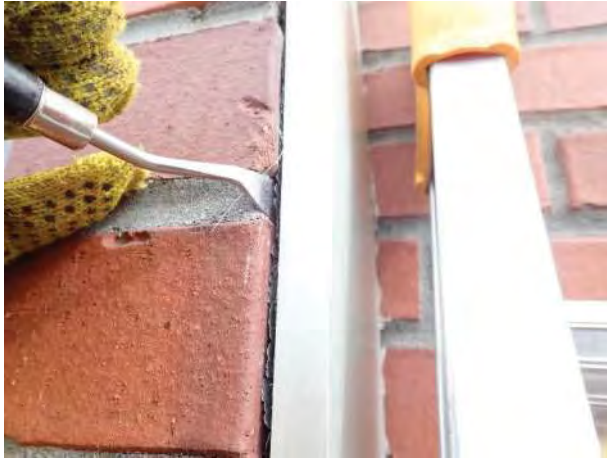
Photo No. 81 - View of what appears to be the edge of the flexible flashing, just visible under the decorative aluminum archway cladding panels. The membrane has degraded and embrittled from having been exposed to UV, weather, and water. Due to the unfinished and deficiently constructed joint, the material is no longer functioning as a through-veneer flashing.
