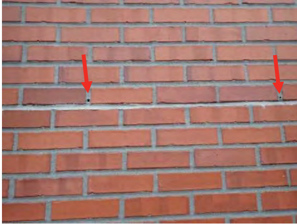
Photo No. 63 - Overview photo of brick veneer weep tubes located approximately every three brick head joints. Many of the weep tubes observed are to be blocked.
