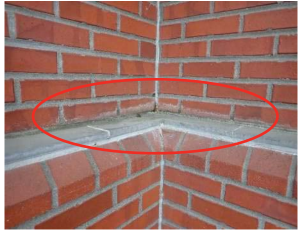
Photo No. 53 - Another view of moisture-related staining at horizontal shelf, at the steel base plate, near the Main Entry at the North Elevation that appears to be holding/ponding and absorbing water.
