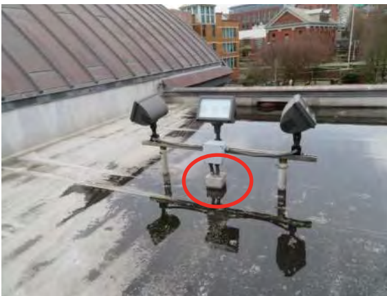
Photo No. 30 - Circle indicates the "pitch pan" type penetration flashing typically present at electrical penetrations at the low-slope roof area. Note that the pan is located in a significant ponding area. One such pourable sealant penetration pocket was observed at each of the eight (8) low-slope roof areas.
