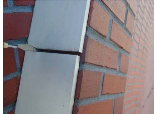
Photo No. 82 - Depicts open decorative aluminum panel-to-panel joint, approximately 5/8" wide, open to water entry to the head of the brick arch. Note flexible flashing was not observed at this location under the decorative aluminum panels, so water and freeze-thaw degradation of portions the brick masonry may occur over time.
