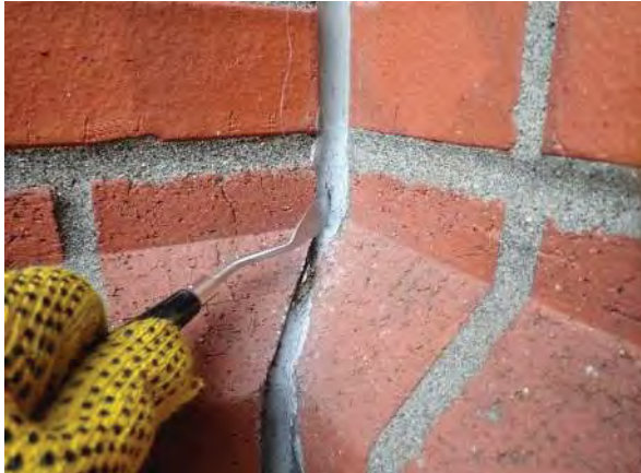
Photo No. 44 - View of flat probe inserted into a cohesively failed sealant joint at brick masonry veneer inside corner expansion joint. This is a typical condition.
