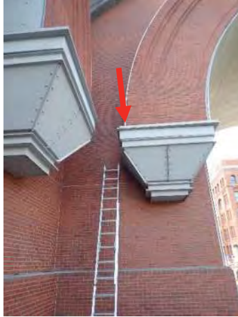
Photo No. 67 - Overview of column bases at main entry and locations of open brick veneer cladding, which should be corrected.
