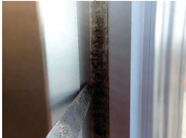
Photo No. 102 - View of interior sealant joint showing signs of repeated wetting and drying, likely from condensation, as evidenced by the dark-colored fungal (e.g., mold) visible on the silicone sealant.
