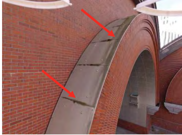
Photo No. 74 - View of large North Elevation archway top as observed from BET&R's drone near the main entry. Note the moss growth promoted by the large open butt joints in the decorative aluminum panel cladding system.
