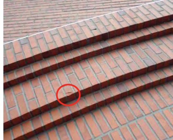
Photo No. 60 - View of spalled brick unit discovered at the South Elevation of the decorative and projecting portion of the façade of the Facility. This spall, occurring along the lower edge (i.e., a drip edge) of the wider/taller/bigger and prominent projecting band of brick is indicative of where water is held along the lower portion of this brick course before dripping off. Any brick that allows that paused water/moisture to permeate into the face of the fired-clay, along the drip-edge of this brick band, may freeze, expand in the frozen clay matrix, and spall or break the face of the brick. This condition is a sign that the previous water repellent has weathered, dissipating, and "wearing out." At this initial spall's depth, of the moisture permeation, it means that it is time to budget for and soon undertake spot repairs, cleaning, and a water repellent project. Please see specific recommendations below.
