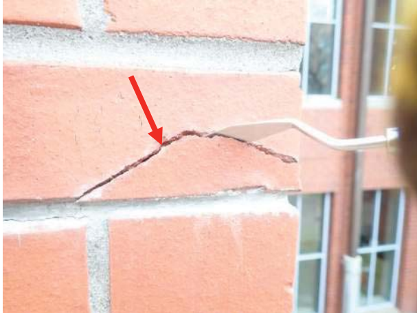
Photo No. 59 - View of fractured brick unit discovered at the West Elevation of the Facility. This type of crack and resultant wide differential separation of the clay brick appears indicative of strain in the wall assembly or floor-line movement. It would be prudent to have a brick masonry-experienced structural engineer review this portion of the facility with BET&R, from the interior and exterior, so as to determine if there is more to a "repair" of the building than just to this isolated portion of the brick masonry veneer. Please see recommendation below for more information.
