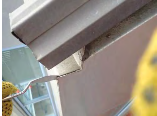
Photo No. 104 - View of open .125-inch thick aluminum panel corner joinery associated with storefront window systems observed at the East Elevation window bay.
