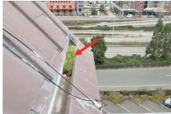
Photo No. 33 - Extensive vegetative growth was observed at several of the membrane-lined built-in gutters, apparently supported by the moisture available due to the gutters' improper slope.
