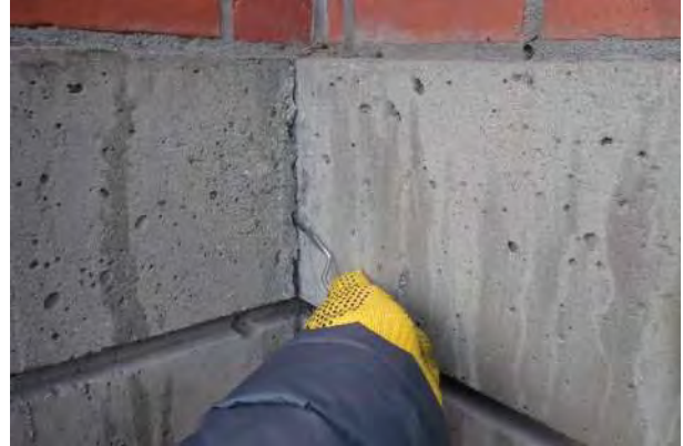
Photo No. 88 - View of open cold joint at inside corner of CIP wall, as observed at the East Elevation, which is susceptible to water migration and freeze-thaw spalling.
