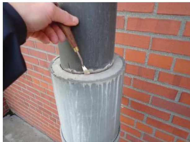
Photo No. 124 - Failed sealant joints at the downspout to below-grade tight-line stub-up connections with wider diameter leader lines were discovered to need replacement while on-site. This was a typical condition, and should receive replacement to avoid freeze-thaw splitting and damage.
