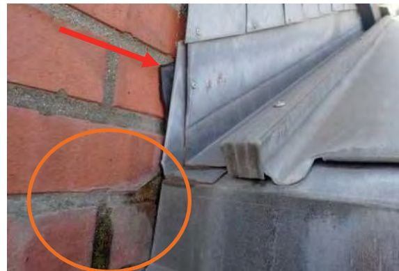
Photo No. 23 - Photo depicts opening between the sheet metal roof-to-rising wall flashing and the brick veneer at the North Elevation of the Anthem Café Dormer. A small portion of the underlying self-adhering ice and water protection membrane is visible at the incomplete termination of the sheet metal roof-to-rising wall flashing (arrow). Water was also observed to be on the brick behind the flashing at this location (circle); these roof-to-wall transition flashings need to be retrofit.
