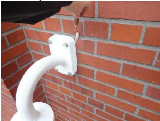
Photo No. 50 - Depicts flat probe inserted behind light fixture base mount at brick veneer, which is open to water entry and leak water migration into wall system.
