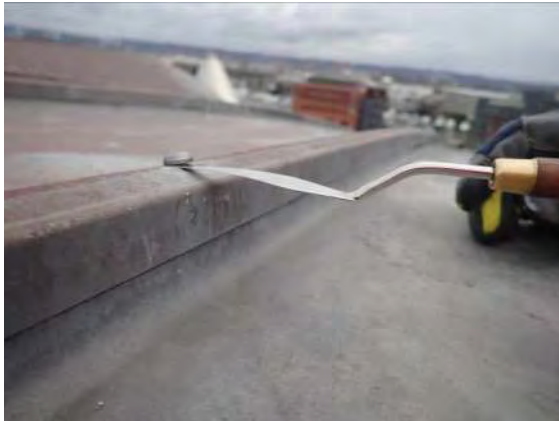
Photo No. 14 - Photo depicts roof technologist's tactile probe inserted between the head of the loose stainless steel screw fastener and the lead-coated copper roof panel seam battens at the apex of the steep-slope barrel roof area on the southern (i.e., windward) portion of the building.
