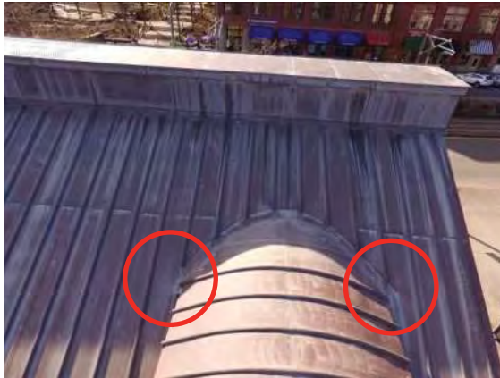
Photo No. 18 - Photo depicts overview of the apex flashing at the dormer roof-to-main roof transition at the east side of the Anthem Café portion of the facility.
