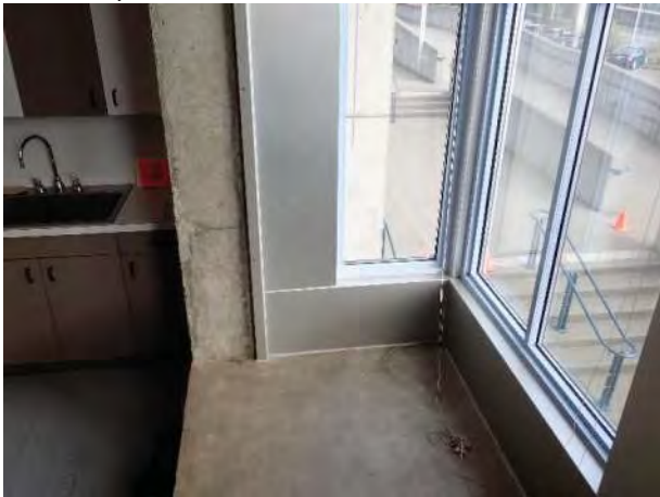
Photo No. 101 - View of interior of Bay Window at East Elevation, and location of residual moisture staining at the interior likely from the reported repetitive condensation occurring at these units.
