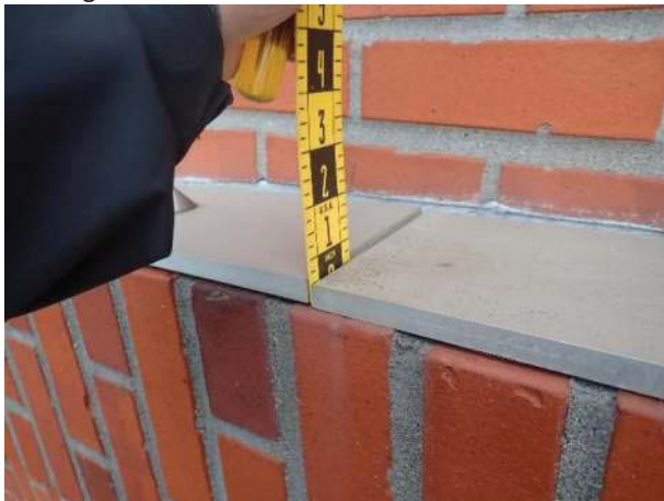
Photo No. 83 - Depicts open decorative aluminum panel-to-panel joint, approximately 1/2" deep, open to water migration to the head of the brick arch. Note that flexible flashing, nor an underlying back-up metal flashing that could and should have lapped out over the outer edge of the brick to protect the masonry from freeze-thaw damage, was not observed all along this area under the decorative aluminum panels.
