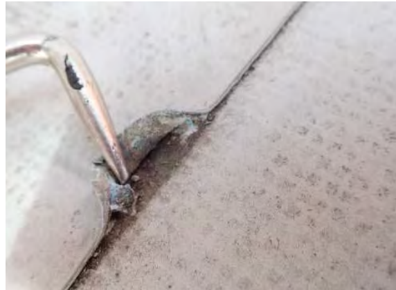
Photo No. 29 - Depicts open and disbonding membrane seam at the southeast corner roof area. Disbonding, or partially disbonded seams were observed in a few select locations, primarily at the west side of the southeast corner roof area.
