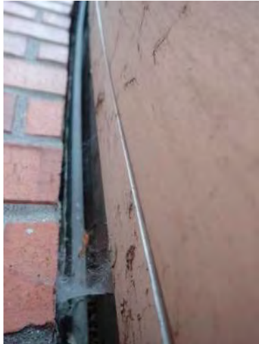
Photo No. 77 - Depicts large gap, approximately 1-inch + at this archway panel-to-brick veneer ledger angle intersection. It appeared that a flexible self-adhering flashing was applied to “flash” the void, however, the flashing membrane is currently unadhered, open, and exposed to UV degradation, and the intersection is wide open to wind-driven rain and migratory water – on both sides of the steel ledger angle.
