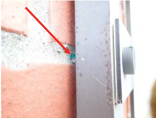
Photo No. 48 - View of typical bolted connection at signage anchor for the Anthem Café is open to leakage and water migration in to the wall.
