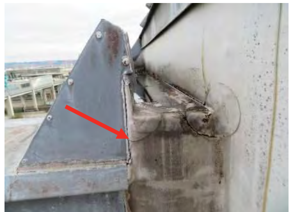
Photo No. 35 - Arrow indicates vulnerable and open intersection between existing membrane gutter liner and the sheet metal end-closure flashing. Water appears to be able to drain out of the end of the gutter and intrude into this open and unsealed transition. These details should be corrected via their redesign by a roofing-experienced and knowledge roof consultant, assisting the architect, for the upcoming reroofing project design phase.
