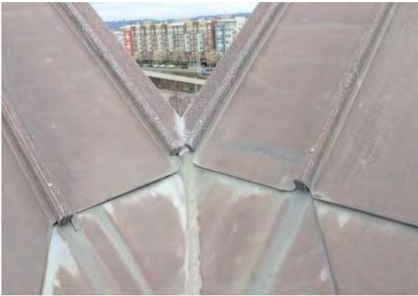
Photo No. 4 - Depicts the intersection of the steep-slope roof perimeters and specifically the rake edge roof panels at the intersecting sheet metal roof areas. The sealant applied at the laps of these sheet metal roof panels and flashing components has degraded and reached the end of its useful service life.
