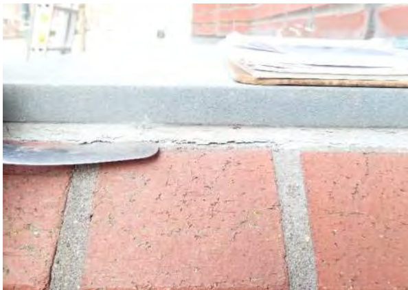
Photo No. 46 - Depicts flat probe inserted into an adhesively failed sealant joint below steel plate at column base location. This is a typical condition.
