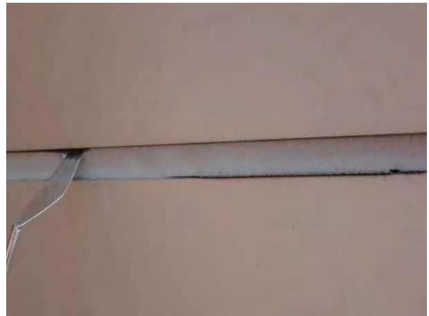
Photo No. 116 - Depicts one of the locations where the soffit panel joint sealant is adhesively failing off of one or in some places both bond-faces, and is in need of spot replacement.
