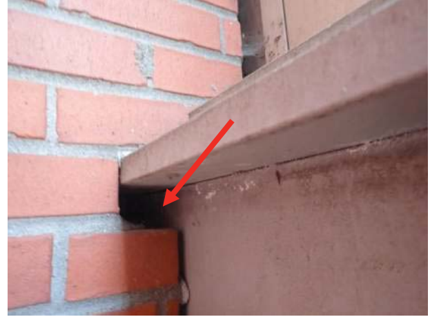
Photo No. 68 - View of large open gap and unsealed joint along at C-Channel penetration through brick veneer at base of archways near Main Entry Area. This location should be closed with partial brick, properly mortar-set, then a backer rod and sealant joint installed between brick and steel member.
