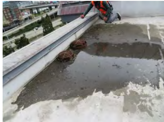
Photo No. 39 - Photo depicts significant buildup of silt and organic debris, as was typically observed at low-slope roof areas.
