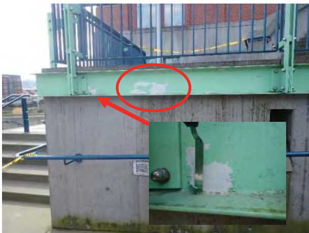
Photo No. 123 - Locations of paint coating peeling and disbondment at hand railings and related steel fascia and connections were observed adjacent the Main Entry plaza of the Museum facility.
