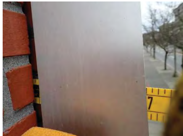
Photo No. 72 - View of ruler inserted under decorative aluminum panel at brick archway and into deficiently left open gap at archway-to-brick veneer wall intersection. The void is susceptible to water migration into the wall assembly, which may be causing hidden degradation and damage to underlying components.
