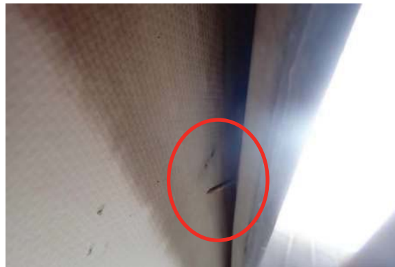
Photo No. 37 - The lower portion of the sheet metal counterflashing was apparently intended to be secured via engagement into/with a concealed stainless steel continuous cleat. BET&R observed that at numerous locations the cleat was either not effectively engaged with the counterflashing’s hem, or the cleat was itself displaced due to insufficient securement with smooth-shanked copper nails (circled), or both.
