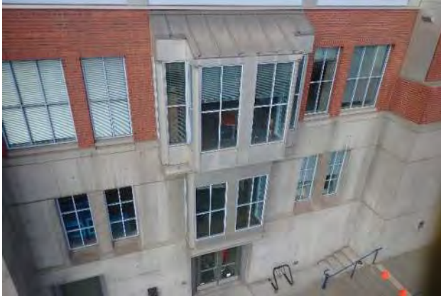
Photo No. 99 - Overview of protruding window bay at the East Elevation, which is a reported area of fairly intense condensation issues with respect to the aluminum framed window system.
