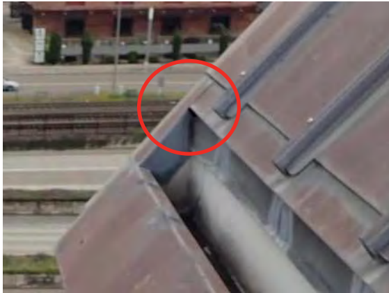
Photo No. 12 - Photo depicts opening at the sheet metal eave edge flashing-to-membrane gutter intersection. The unsealed termination of the roofing membrane was observed to be exposed at this opening, which is in need of correction.
