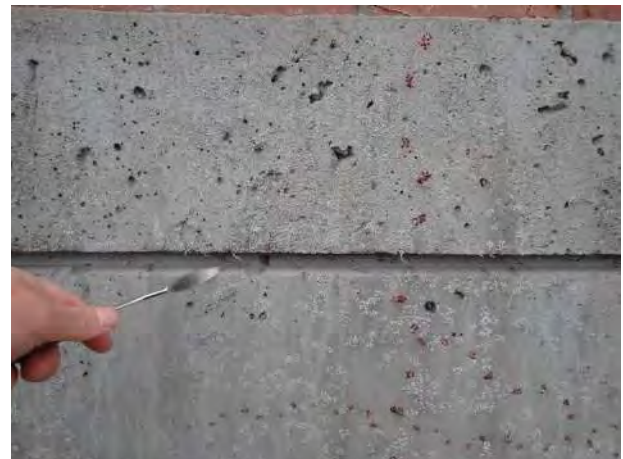
Photo No. 86 - View of “bug holes” and rock pockets, which were not sacked & patched during original construction, are visible and holding some organic growth as observed at the CIP walls. This condition is not necessarily problematic provided the concrete receives an appropriate cleaning and proper application water repellent (including within the voids) at regular intervals as the concrete ages. If the wall were thoroughly cleaned, the voids could be grouted/filled with an appropriate color-matching cementitious grout or repair material if desired.
