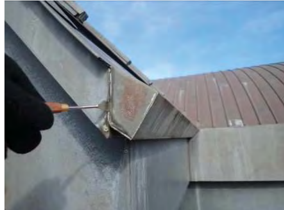
Photo No. 17 - Photo depicts roof technologist's flat metal probe carefully inserted into the failed and open sealant at the sealant-dependent sheet rake edge-to-sheet metal gutter flashing intersection. Due to anticipated rain water runoff migrating into these open joints, BET&R recommends including this failed detail in to an upcoming roofing and flashing repair & retrofit project, which BET&R would be glad to assist SSWA and the Museum to design and see to completion this year as needed.
