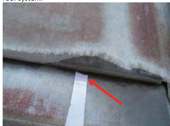
Photo No. 21 - Water-finding paper indicates that moisture is present, emanating from this sheet metal intersection. The upslope deficient detailed conditions should also be included in an upcoming roof repair and retrofit project, so that they can be carefully re-designed and retrofit to keep wind-driven rain and water from entering the roof for long-term successful performance of the roof system.
