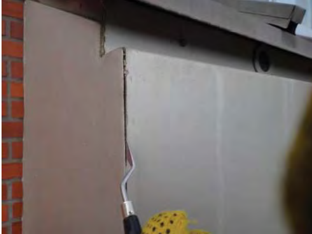
Photo No. 103 - View of open .125-inch thick aluminum panel end-joinery associated with storefront window systems, as observed at the East Elevation window bay.
