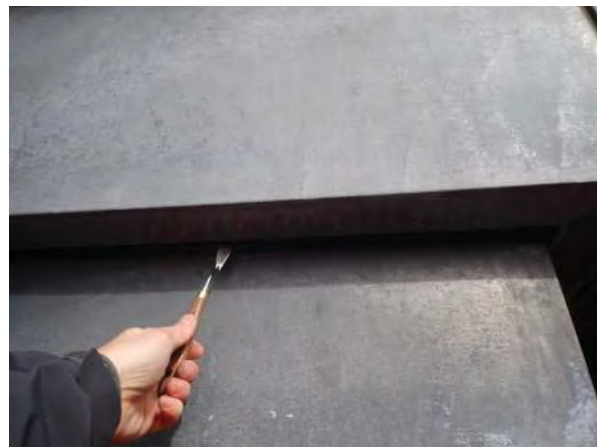
Photo No. 112 - Depicts a tactile flat probe inserted into failed silicone sealant joint at the underside of the break of the cornice element, which is segmented and installed in sections. The majority of the sealant appears to be in good shape, but spot repairs are needed.
