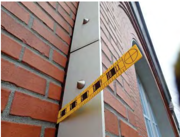
Photo No. 71 - View of Building Envelope Technologist's high-vis ruler, carefully inserted into open gap at archway-to-brick veneer wall intersection. This large gap is susceptible to water migration and leakage into the cladding system.
