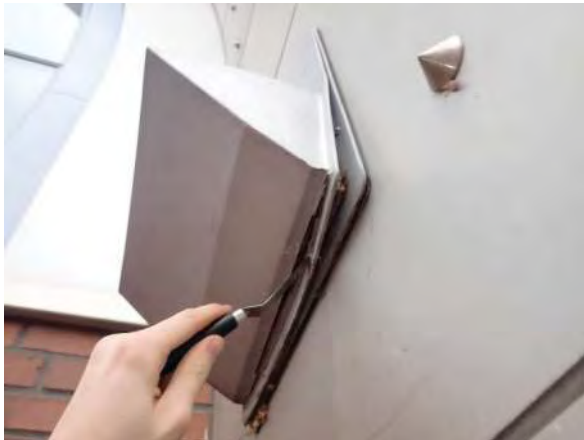
Photo No. 117 - View of displaced light fixture in need of re-securement and weatherproofing retrofit attention.
