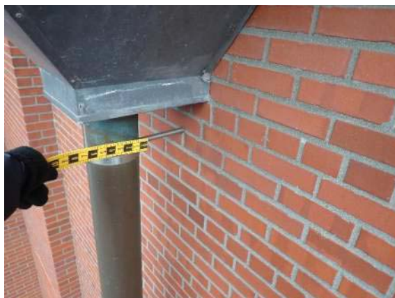
Photo No. 43 - Depicts 6-inch downspout typically observed at drain locations.
