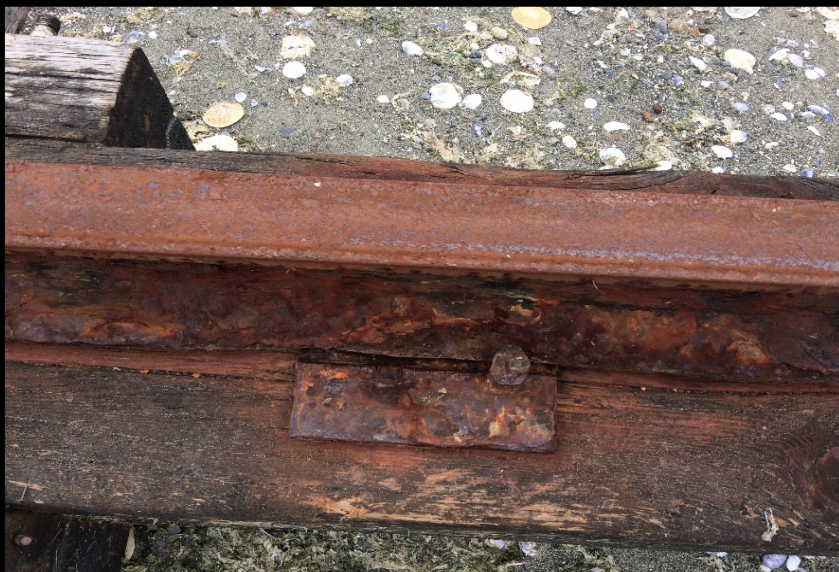
The fasteners have corroded and are failing.
