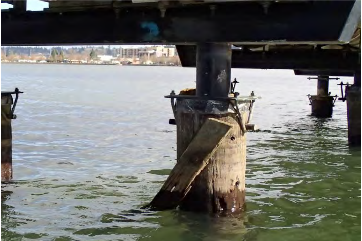
Photo 3 - Typical abandoned bolt holes in piling and section loss in bracing member
