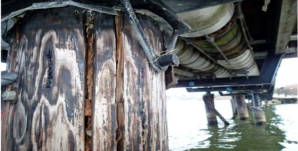
Photo 1 - Example of Rotten Pilings - Pile 7C is badly split with internal rot at the top
