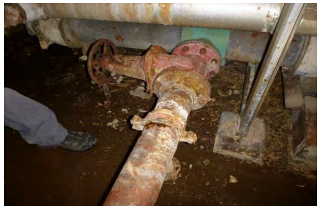
Figure 2: Aged Steam Distribution System
