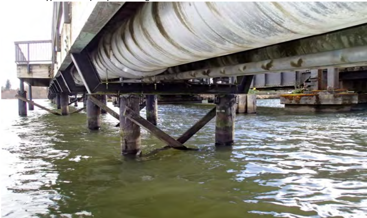
Photo 4 - Typical two-pile pier configuration
