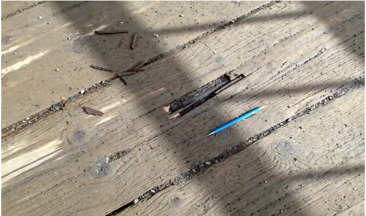
Photos 5 & 6 - Rotten Deck Boards-from above and below
