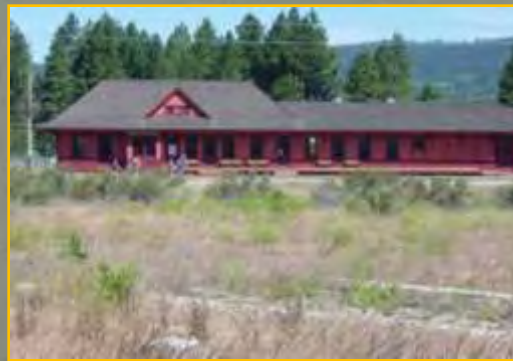
Rehabilitation of historic Cle Elum train depot used sustainable practices
