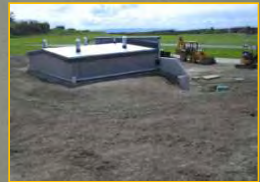
Green Roof used for Fort Casey comfort station
