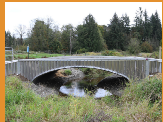
Removing fish barriers and replacing them with bridges that allow fish access.
