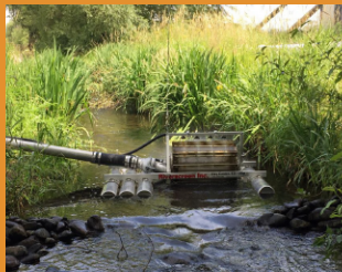
Installing fish-friendly screens on irrigation intakes.
