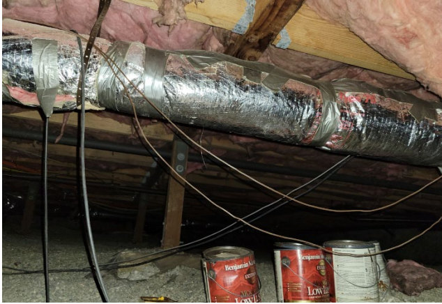
Crawlspace and Ductwork Below Office Area
