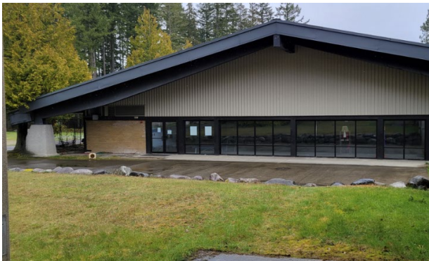
Recreation Building Facing Pool
