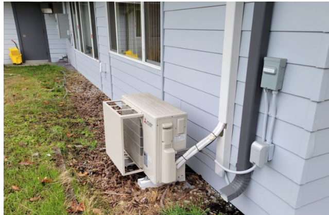
Server Room AC Unit Outdoor Section
