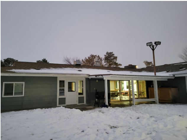
Sunrise Community Facility Note: Air Intake and Kitchen Exhaust Fan
