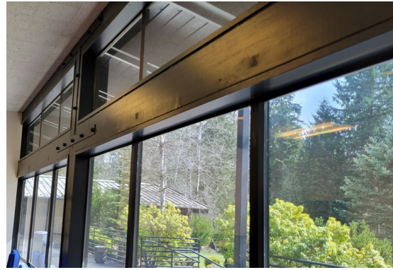
Typical Single Pane Windows
