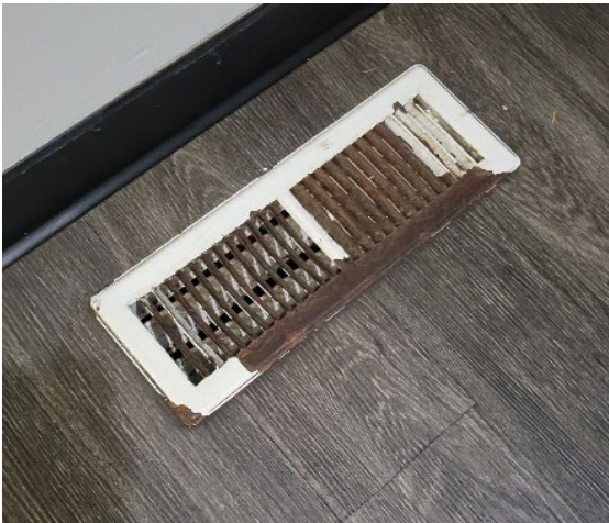
Floor Register near Entry
