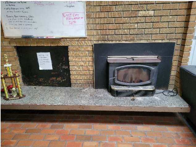
Wood burning stove and wood pass-through door
