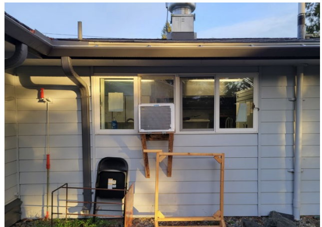
Kitchen from Exterior
