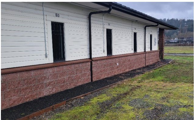
Exterior view at sleeping rooms
