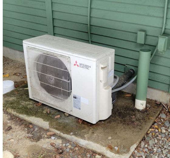
Server AC Outdoor Unit
