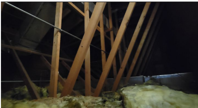
Ceiling Space above classrooms
