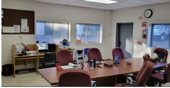
Break Area. BMS Computer on Far Wall
