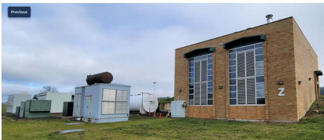
Central Plant Building
