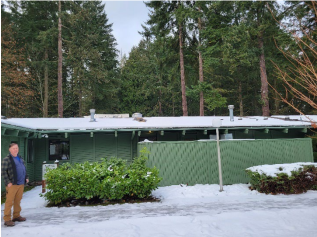
View of Facility from Parking Lot
