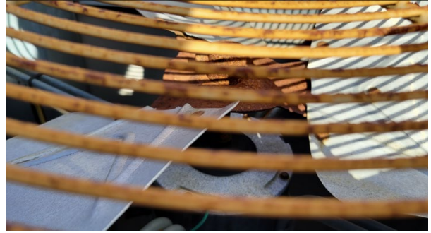
Condenser unit for AHU-F2
