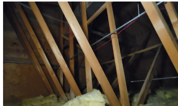
Ceiling Space above classrooms
