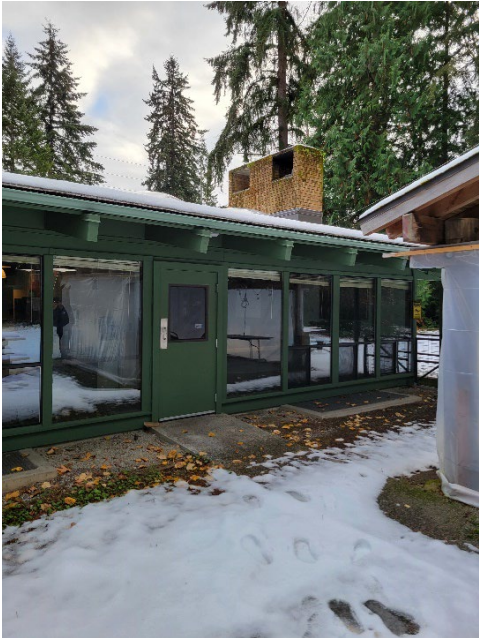
Exterior view of common room from rear courtyard
