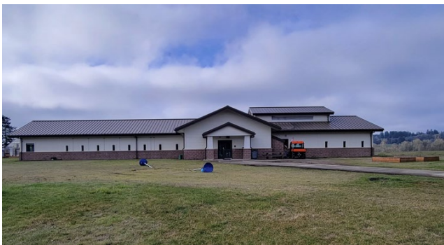
Cedar Building "C"
