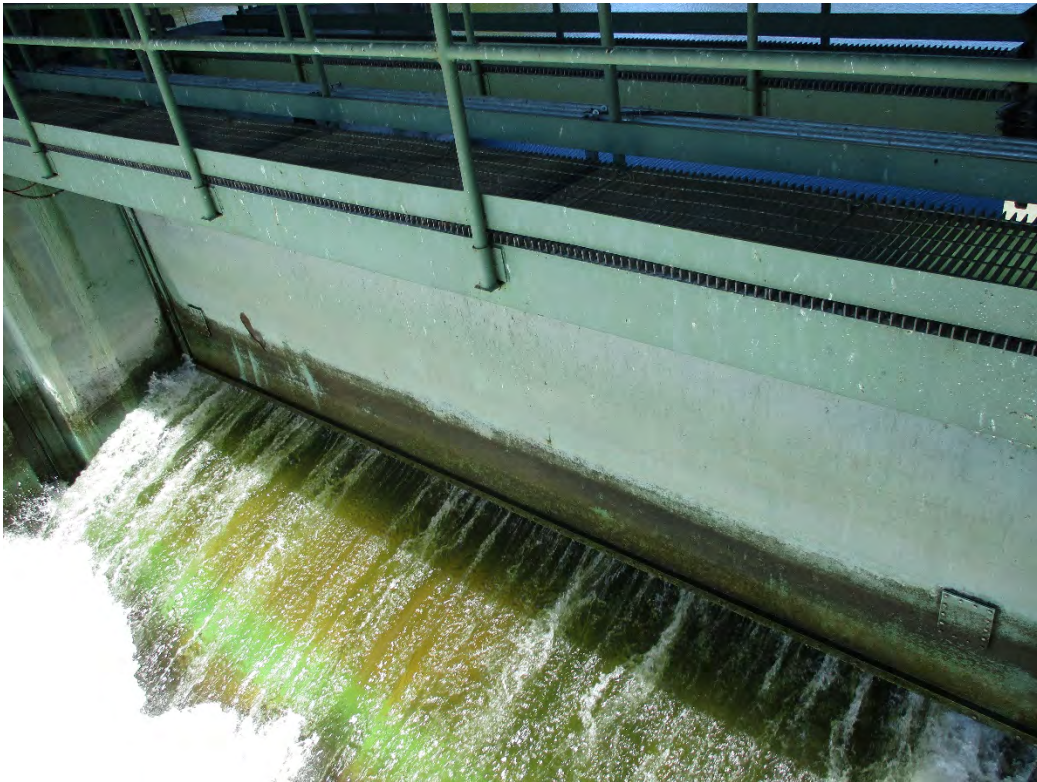
Figure 13 – Gate #3 (from downstream)
