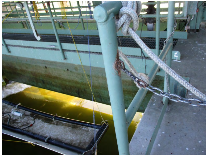
Figure 9 – Gate #1 Fully Open (from upstream)
