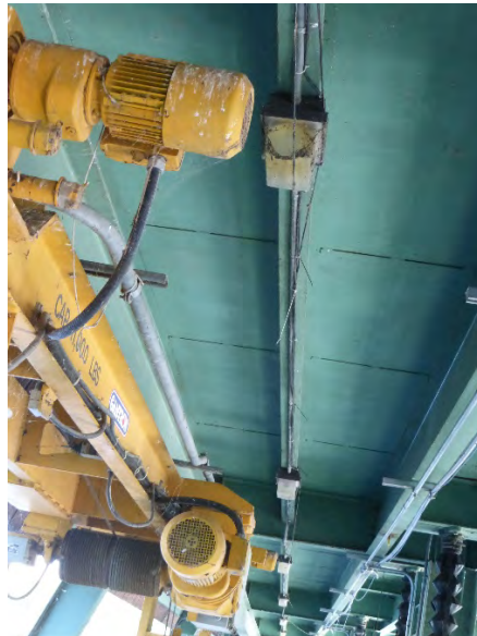
Figure 26 – Existing Dam Outdoor Ceiling Lights
