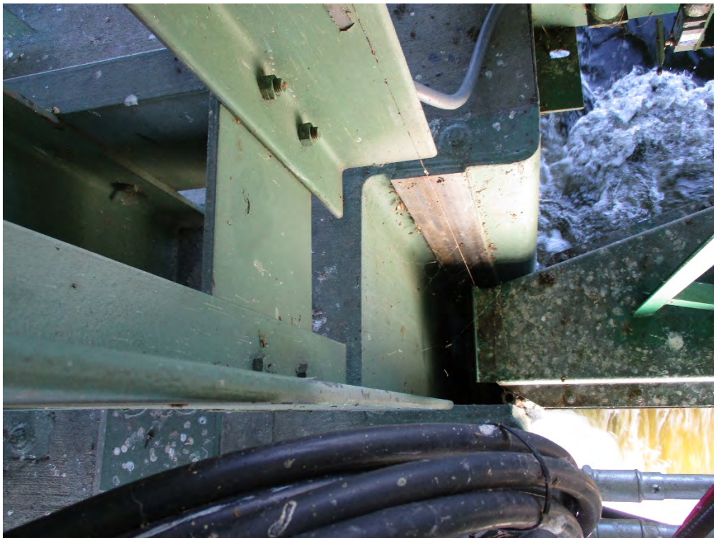
Figure 14 – Gate #3 Slot and Gate
