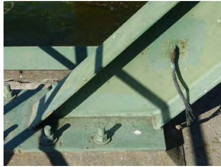
Figure 31 – Grounding Cable Exothermic Welded to Structure
