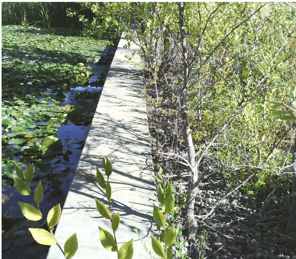
Figure 36 – Looking Upstream Along the Upstream East Bank Wall
